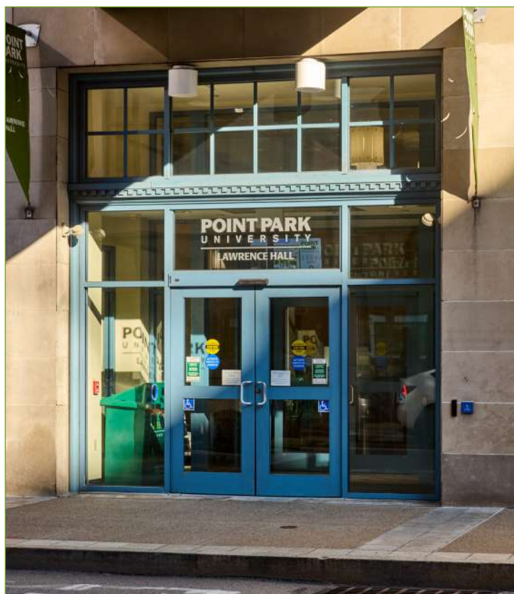
Caleb McCartney | The Globe The Wood Street entrance of Lawrence Hall and the grate creating the alleged source of the "sewage" smell when the doors open.
